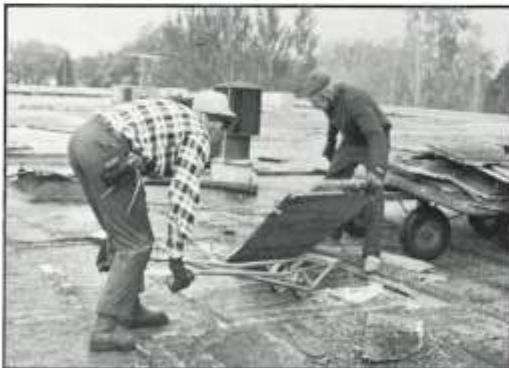
PRY ROOFING UP
