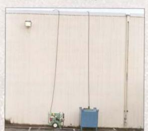
Material and pump stay on the ground with the 55-gallon drum or bulk tote. Material is pumped up to the roof through a hose.
