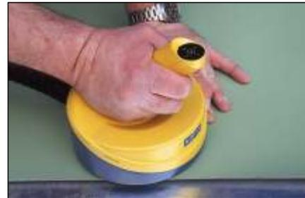
4. Remove Centrix tool and apply magnet to welded plate. Leave magnet in place 40-50 seconds until weld is cool.
